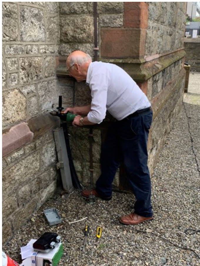
Noel making holes through 3 foot thick walls
